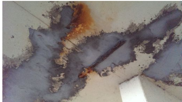
Corrosion in reinforced concrete near sea defences.
