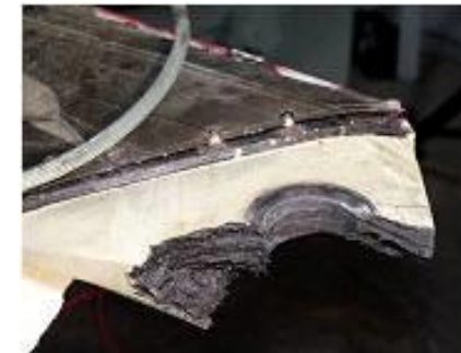
Fractured strut on AA587 stabiliser
